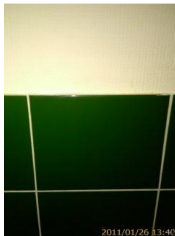
All Walls in Room Wall finish
