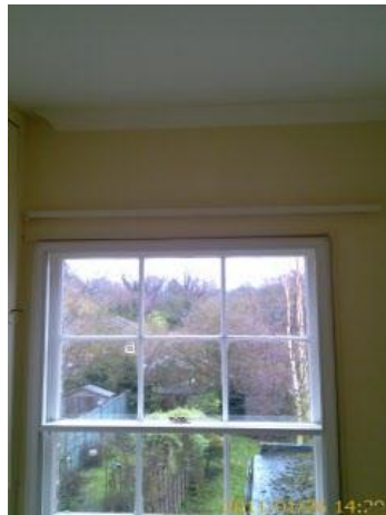
All Windows in Room Window frame/sill, Window glass, Curtain Rail
