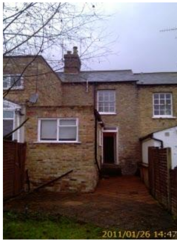
Rear of building
