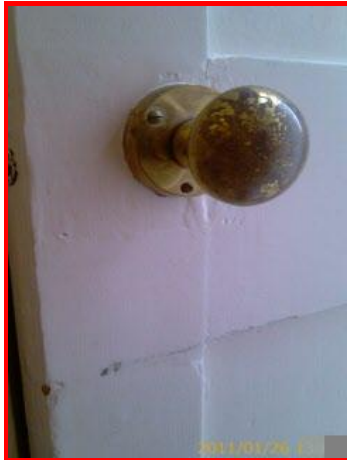
Door to stairs
