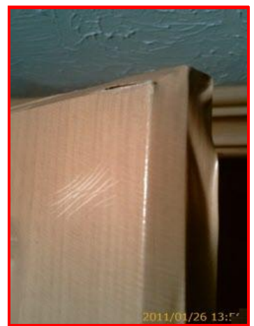
Kitchen unit - eye level - scratched, Kitchen unit - eye level - melted (from misuse)
