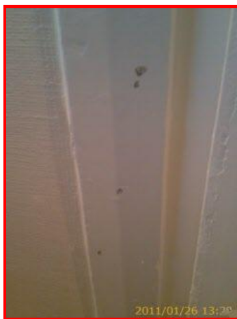
All Doors in Room Door frame - marked
